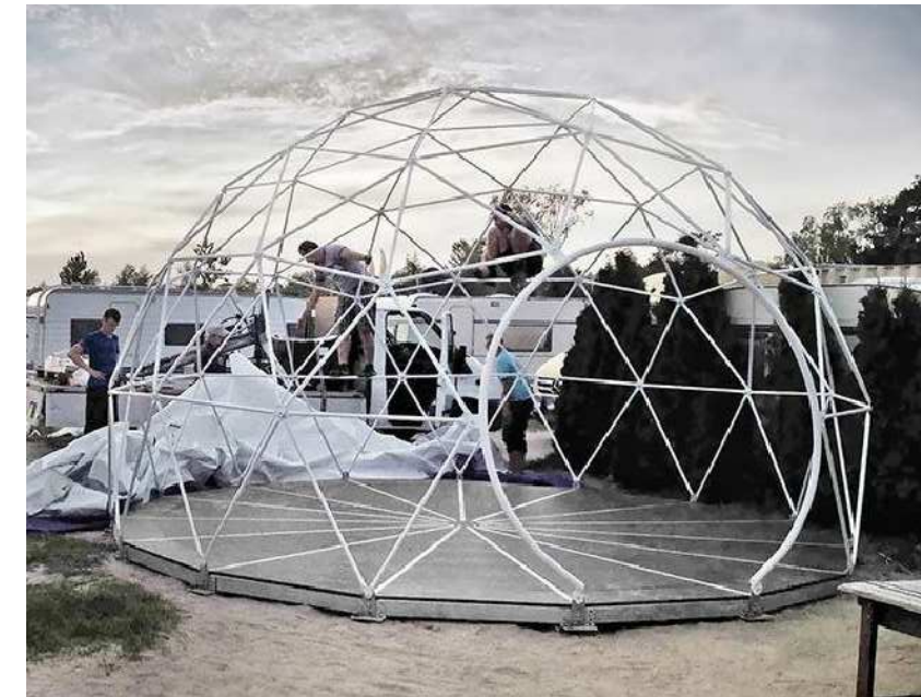
ASSEMBLY FRAME / FLOOR VIEW
